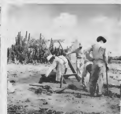
PUBLIC WORKS team, digging near surface on Arends farm. EQUIPO DI OBRAS PUBLICAS cobando den cuencu di Arends.
